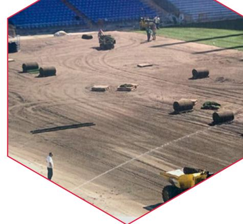
A new mixed surface is installed, blending natural grass with 17 million synthetic fibers.
